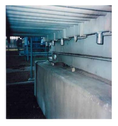
Typical transformer radiators have a half coupling with a plug installed, located on each radiator bank on the top and bottom to facilitate draining individual radiators. These are prone to leak; Colt service trucks stock several sizes of custom repair caps that are installed over the active leak and then are injected with our S-22 sealant to stop the leak.
